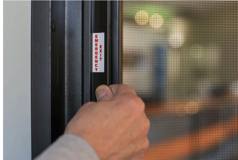
Egress screens are easily opened using the panic bar.
