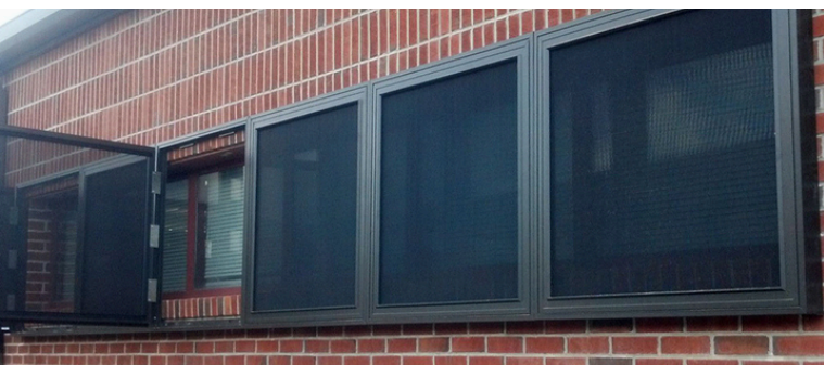
Egress screens installed on back, ground level windows per code.
