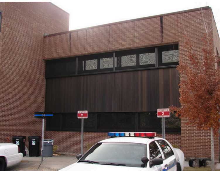
Fixed Screens protect upper levels of precinct.
